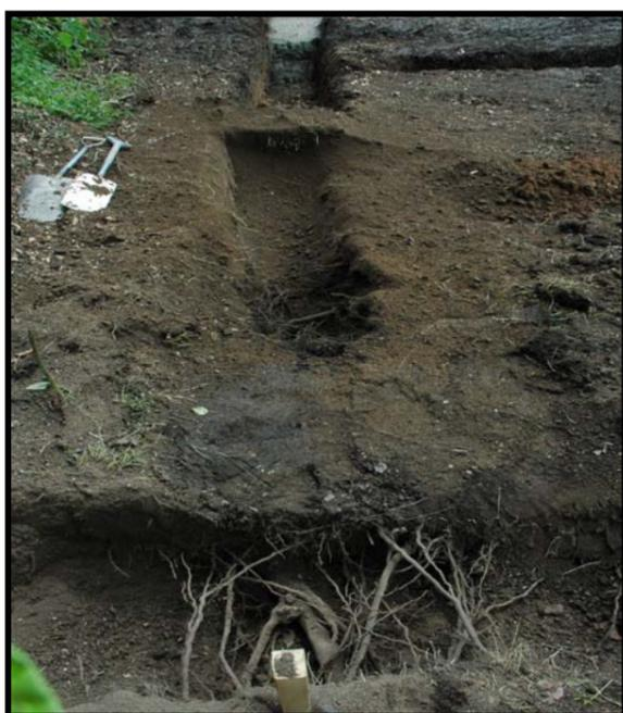
Where it becomes necessary to excavate a trench close to or under the canopy of a tree, these tools can be used to expose roots that may then be either bent out the way of the trenching work or cut back using target pruning. This reduces the stress caused to trees by preventing roots being ripped out the ground by a mechanical excavator, therefore prolonging the trees life expectancy and enabling the retention of trees that may otherwise have been removed.
